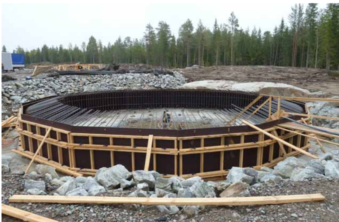
Image 3. Wind turbines are huge constructions. For example building the foundations takes about 600 m 3 reinforced concrete. Also the installation field and other infrastructure built for the wind turbines changes the natural environment greatly especially in sensitive arctic hilltop areas. Photo: Timo Jokelainen.
